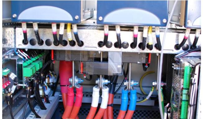
*Three phase cable connections to the bidirectional inverter and sensors*
